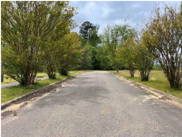
Photo 3 Paved roadway onsite
