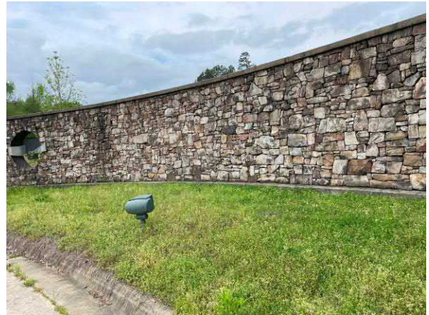
Photo 2 Rock wall on east side of site
