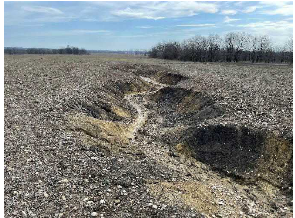
Photo 4 Erosional ravine on mid-south portion of property
