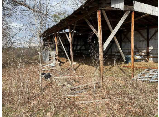
Photo 2 Deconstructed barn south of South Wood Road
