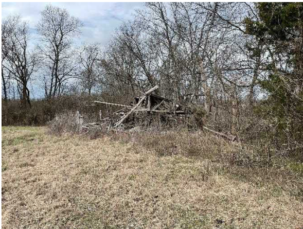
Photo 11 Demolished shed on east edge of site
