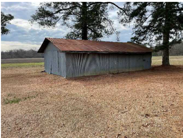
Photo 5 Barn at the intersection of S. Wood Rd and W. Reynolds Rd
