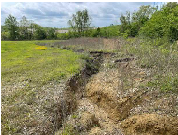
Photo 5 Drainage on western portion of site
